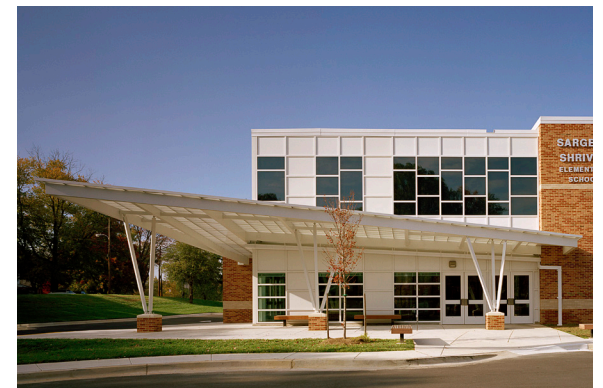
Sargent Shriver Elementary School Silver Spring, MD | Architecture Inc
