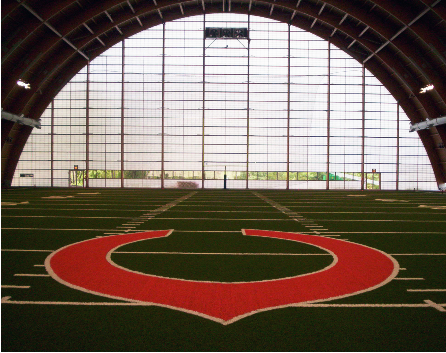
Walter Payton Center: Chicago Bears Indoor Practice Facility Lake Forest, IL | Lohan Caprile Goettsch
