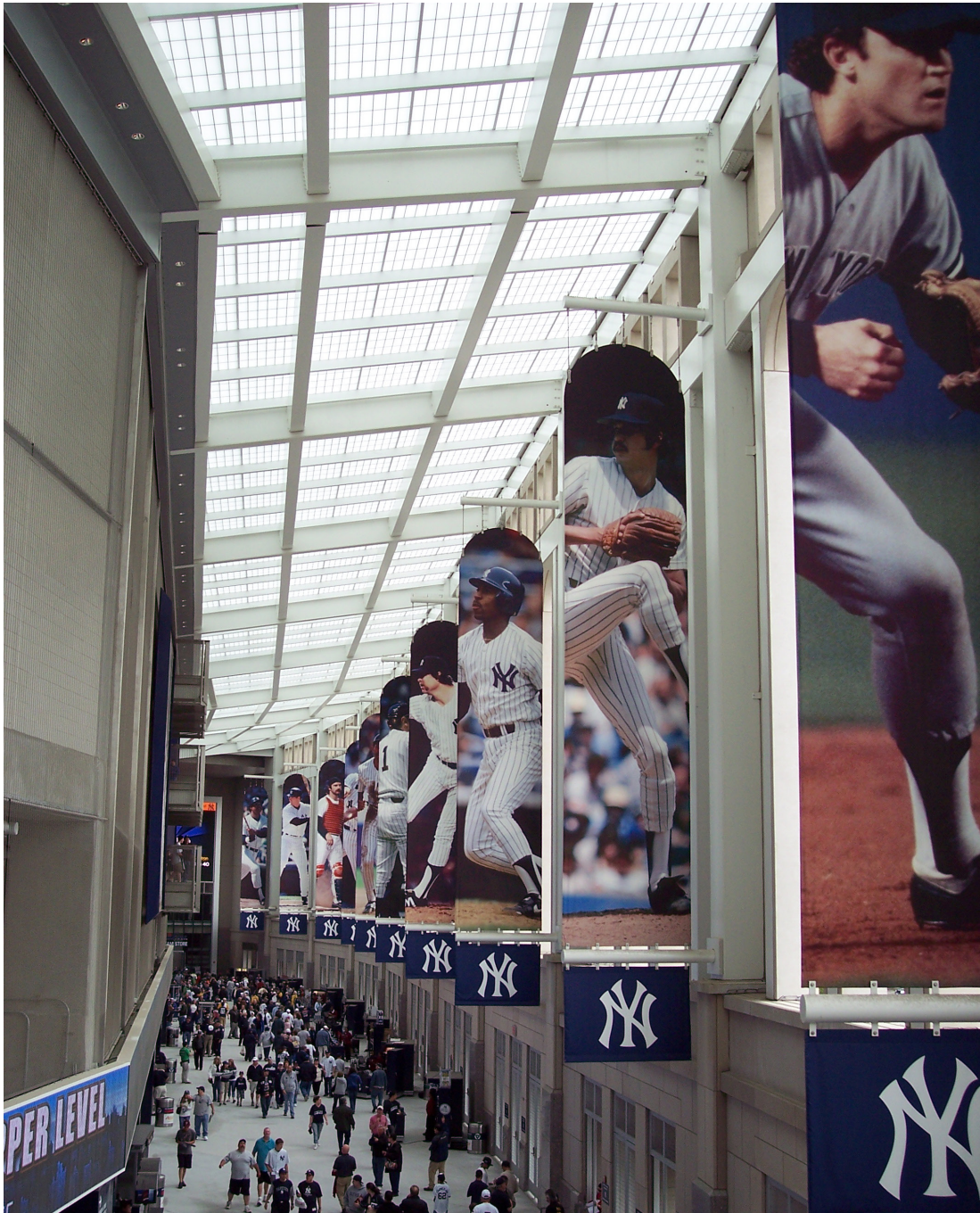
Yankee Stadium: Kalwall with Clearspan™ System by strategic partner, Structures Unlimited, Inc. Bronx, NY | Populous
