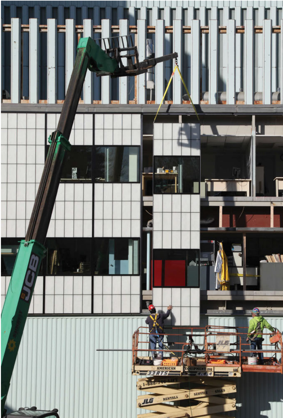
Newington Power Station Newington, NH
